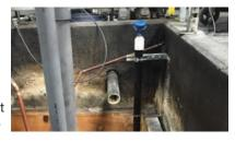
of metals, ceramics and other materials process where process temperatures can exceed 400 degrees. Here, a LG10-0 is installed in a metal manufacturing plant waste sump using a PVC stand pipe to eliminate turbulence. The guided wave sensor is unaffected by the high temperature, condensation and foam.
